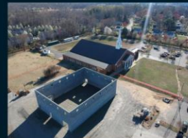
Family Life Center Construction Late 2019
